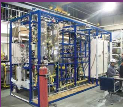
A bio-oil hydrotreating pilot plant
