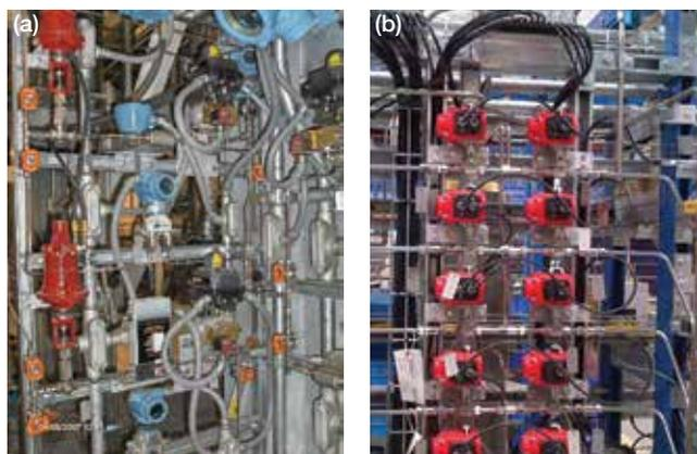
▲ **Figure 4.** (a) Banks of valves and instrumentation installed with metal tubing and electrical conduit are expensive and difficult to alter if additional equipment or connections are needed. (b) Valves connected via plastic air lines and push-type quick-release fittings are less expensive, easier to install and change, and do not compromise safety.
