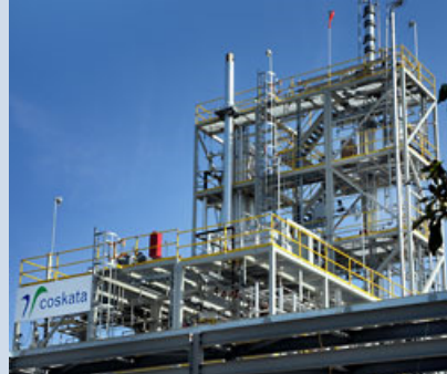
Coskata's cellululosic ethanol demonstration plant in Madison, Pennsylvania, has a production capacity of 40,000 gallons per year of ethanol
